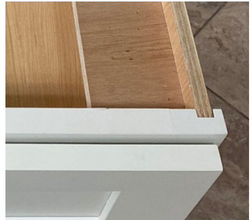
Plywood Box I-Beam Construction
